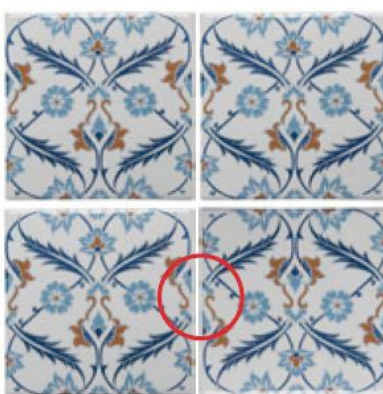
This is incorrect as the patterns on the sides do not line up, because the tile bottom right is upside down
