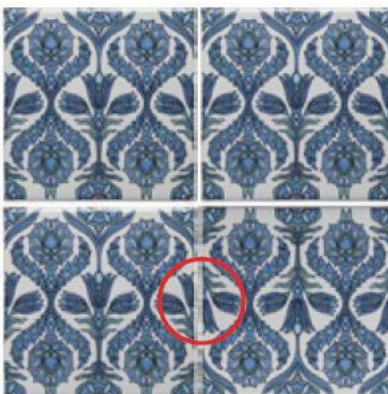
This is incorrect as the patterns on the sides do not line up, because the tile bottom right is upside down
